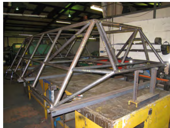
(b) Top Frame fabrication
